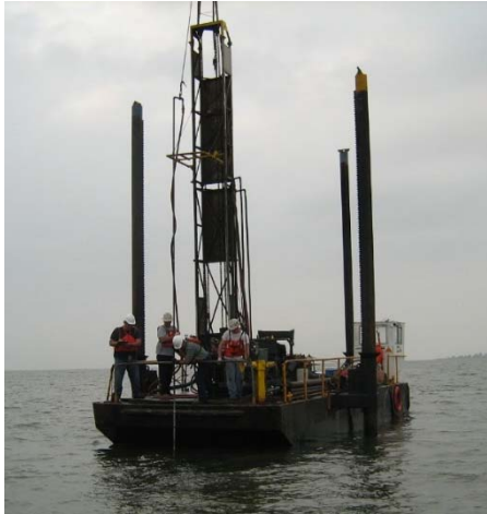
Figure 6-2: Jet Probing
